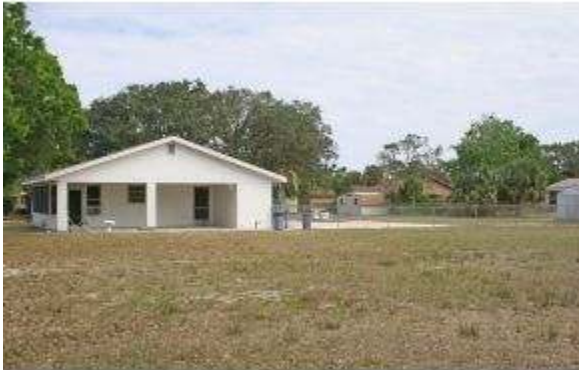
West Side View
